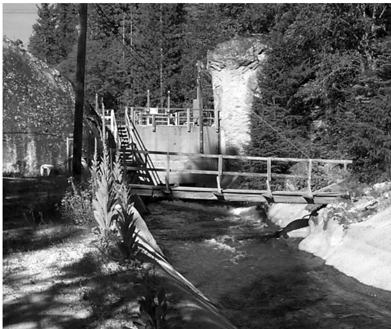
EID (Former PG&E) Canal—Water is pouring in from the diversion dam
