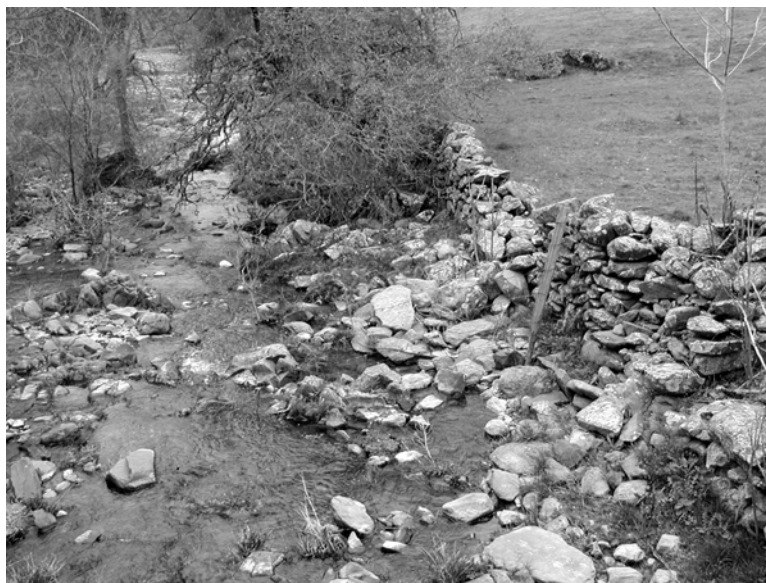
Remnants of rock walls along Carson Creek
