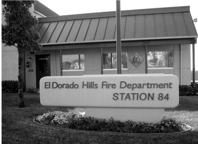
Robert B. Cima Memorial Fire Station on Francisco Drive
