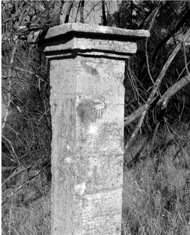
Weathered and vandalized pillar on the Fitch ranch property
