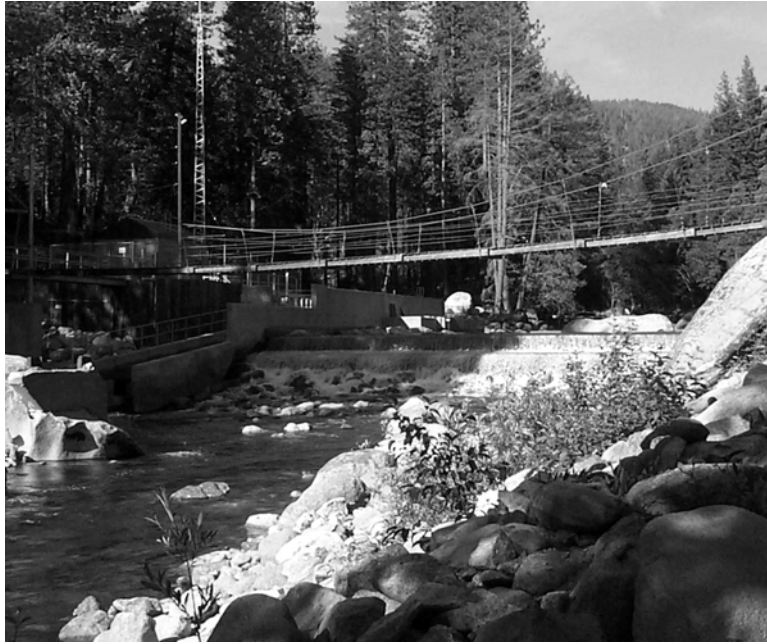
EID (former PG&E) Diversion Dam near Kyburz
