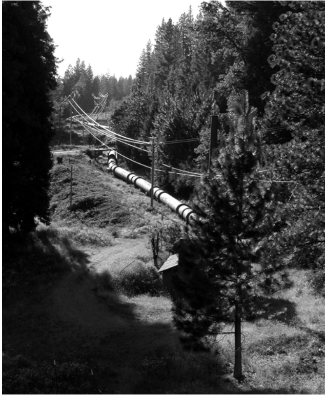
El Dorado Pipeline near Pollock Pines
