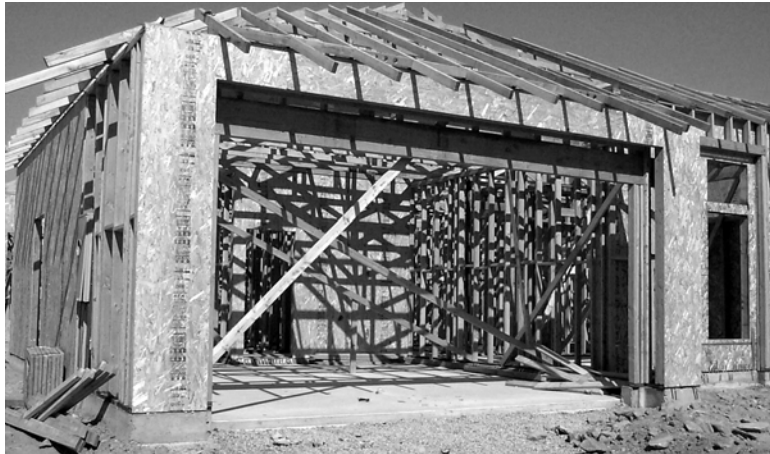
Home construction in Serrano
