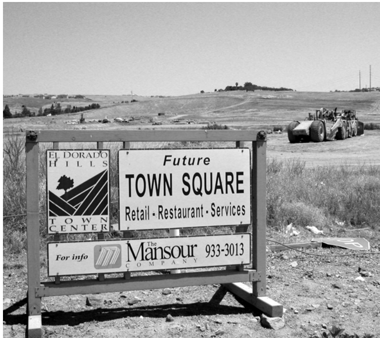
Construction at Town Center East
